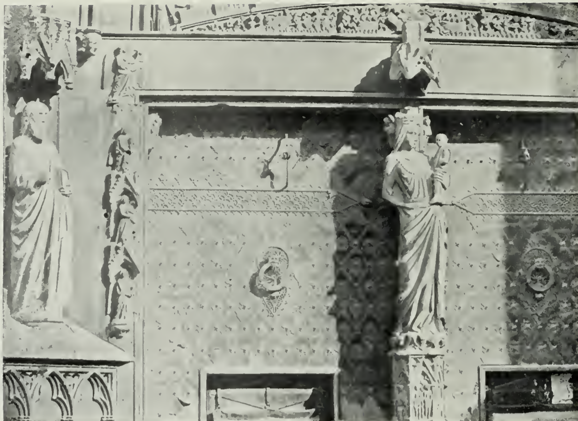
DETAIL OF THE PORTICO, TARRAGONA CATHEDRAL
